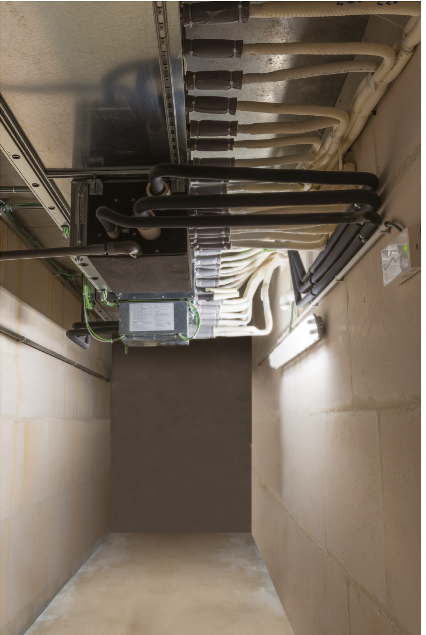
Individual and multi branch selector box installation
