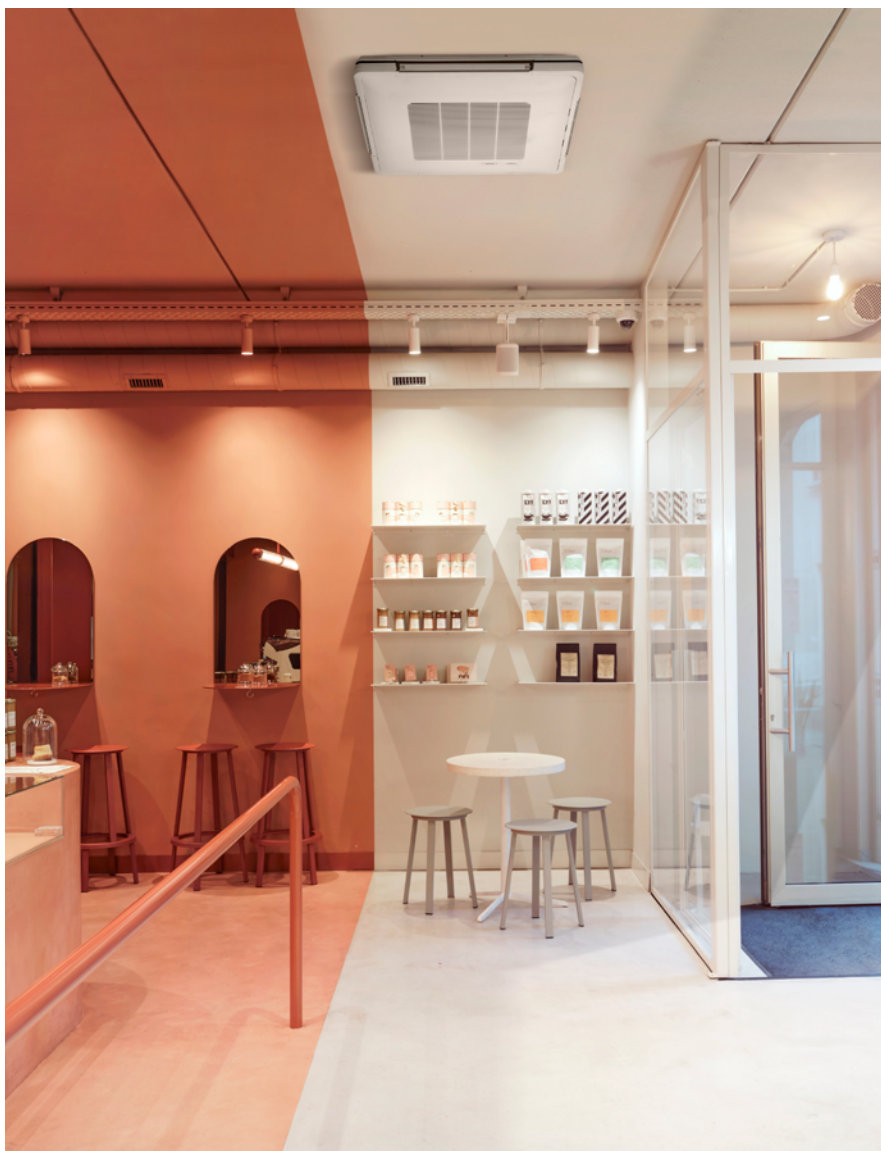
4-way blow ceiling suspended unit
